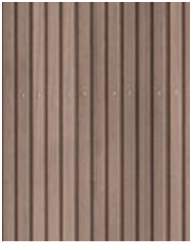
wood cladding in spruce (patio facades) allowed to grey naturally
