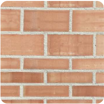
double format bricks 200 x 100 x 110 mm
